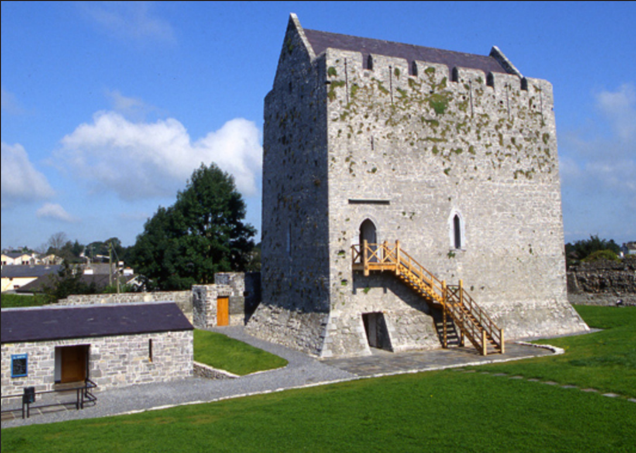
Atheryn Castle in Co. Galway was built around 1250. The Castle consists of a towering keep surrounded by a curtain wall with three towers, one rectangular and two round. The entrance is at the first-floor level. Image courtesy of Dept. of Environment, Community and Local Government.
